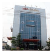
善化保稅倉 Shanhua Bonded Warehouse
