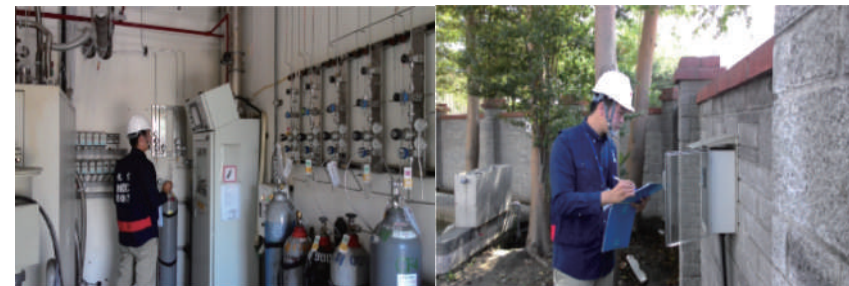
Photos taken during the inspections
